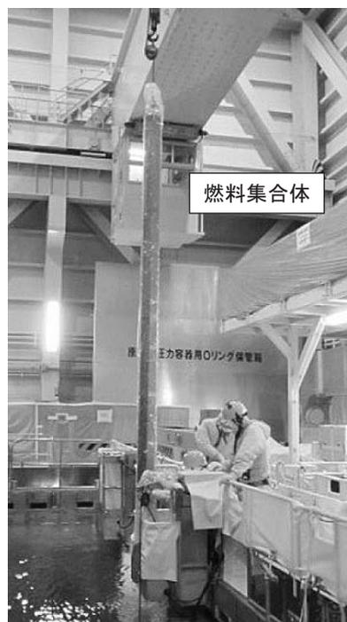
Fig. 2 Lifting a new fuel assembly
